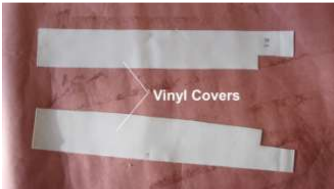
1354. Cut two pieces of vinyl 4" x 18", as shown, and spray the back side with adhesive. Also carefully spray the top frame area with adhesive.
