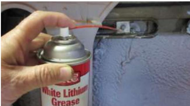
1071. Spray white lithium grease on all accessible moving parts.
