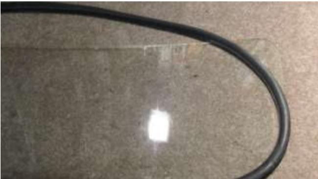
1075. Lay the front seal on the glass according to the final position.
