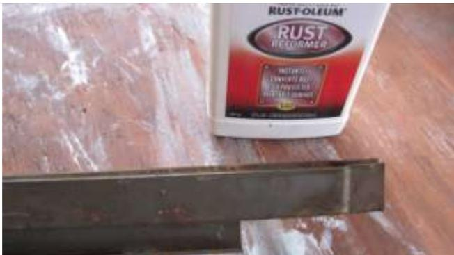
1020. One of the bottom window frames had a little rust on the inside so I applied Rust- Oleum rust remover on the rust area of this frame and let it sit overnight.
