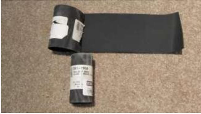
1006. From a new flat roll of molding cut the length to fit into the chrome strips. Make sure it overlaps the width on the outside as shown below.
