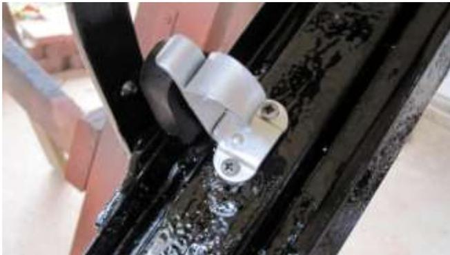
977. Paint the top catch silver and when dry reinstall the catch and rubber bumper on the frame.
