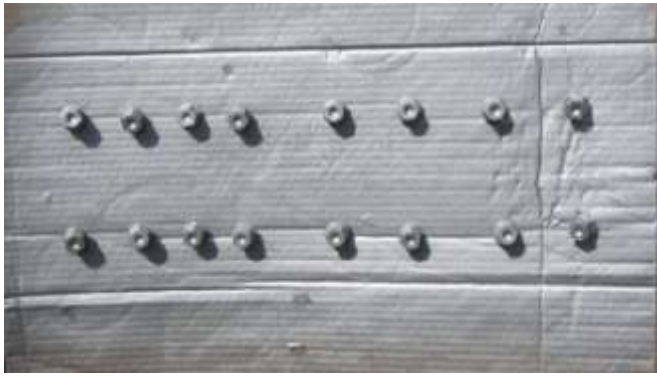
857. The lug bolts were also painted with this color.
