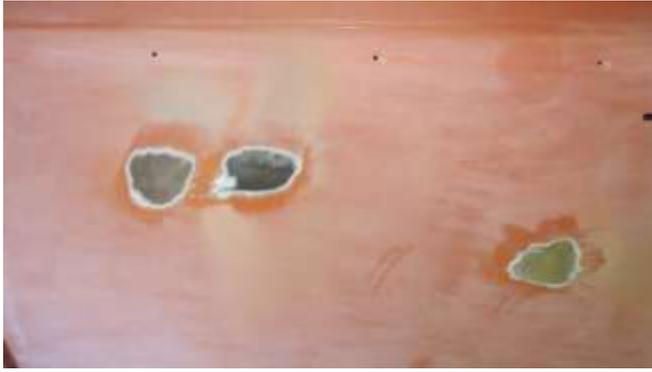
594. Sand the dings down to bare metal with 120 sandpaper, then rough up the bare metal with 80 grit sandpaper.
