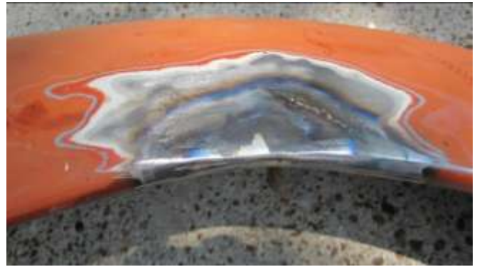
348. Crack, Front side - After
