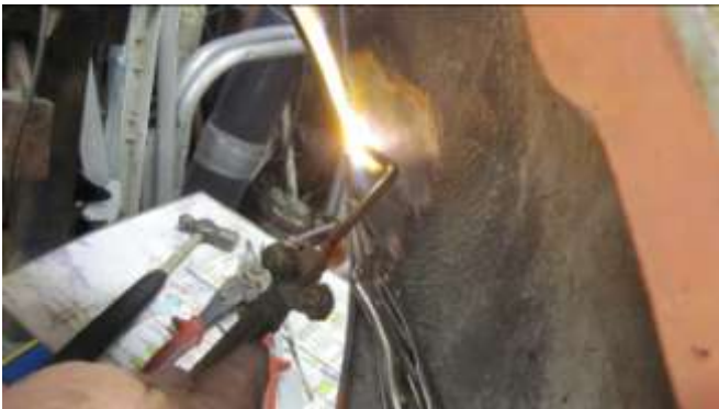
340. Walt, welding the crack on fender.
