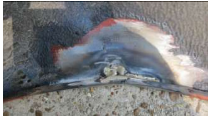
350. Crack, Back side - After
