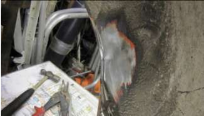
339. Crack after additional cleaning.
