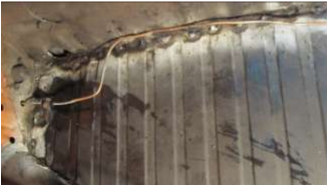
231. Driver's side front: welds completed.
