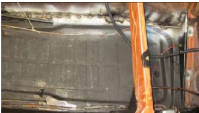
232. Driver's side rear: welds completed.
