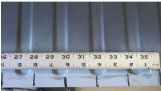
151. Layout lines are on 2 Inches center per the original manufacture specifications per Walt (my welder) directions.
