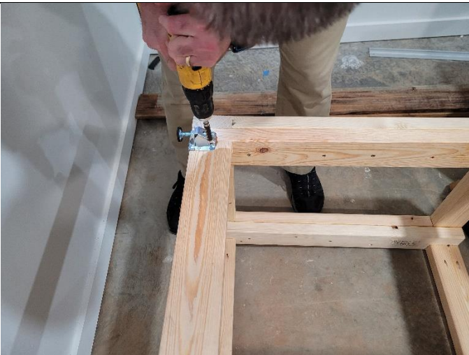
12. Neil installed the leveling feet.
